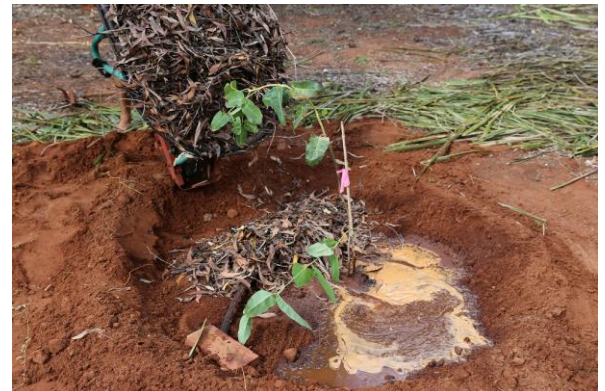
Dig depressions around plants (no lip) over the wet and mulch to trap rainwater and reduce runoff into the bay.
